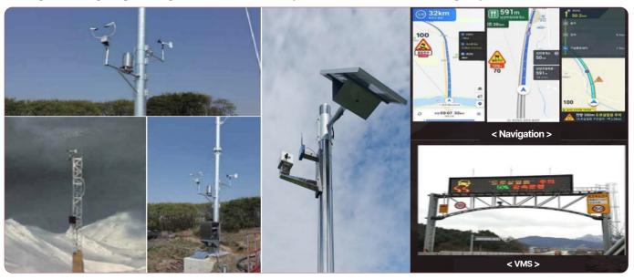
▲ Road hazard weather information (e.g., black ice warnings) analyzed through various sensors installed on highway CCTV poles is provided to drivers.
