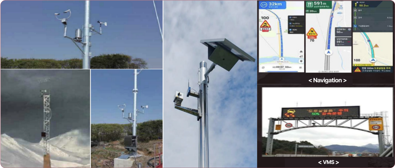
▲ Road hazard weather information (e.g., black ice warnings) analyzed through various sensors installed on highway CCTV poles is provided to drivers.
