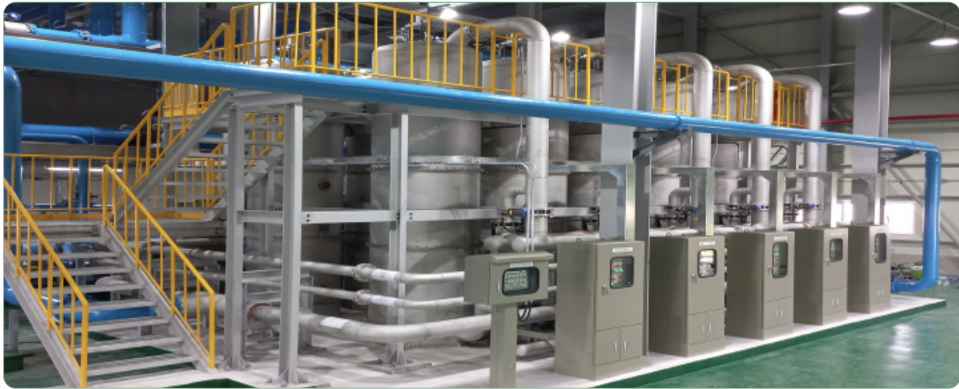
▲ At the Kolon Industries Gumi Plant Water Treatment Center (14,400 tons/day), the fiber filtration system purifies water in just three minutes.
